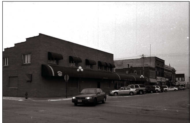
Former Clear Lake Bakery building. Redevelopment of this site was considered a top downtown priority by focus group participants.
